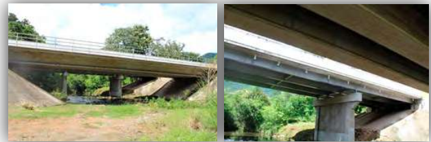
Figures 7 & 8: Pan-American Highway bridge spanning a creek
