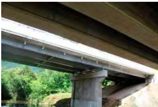
Figures 7 & 8: Pan-American Highway bridge spanning a creek
